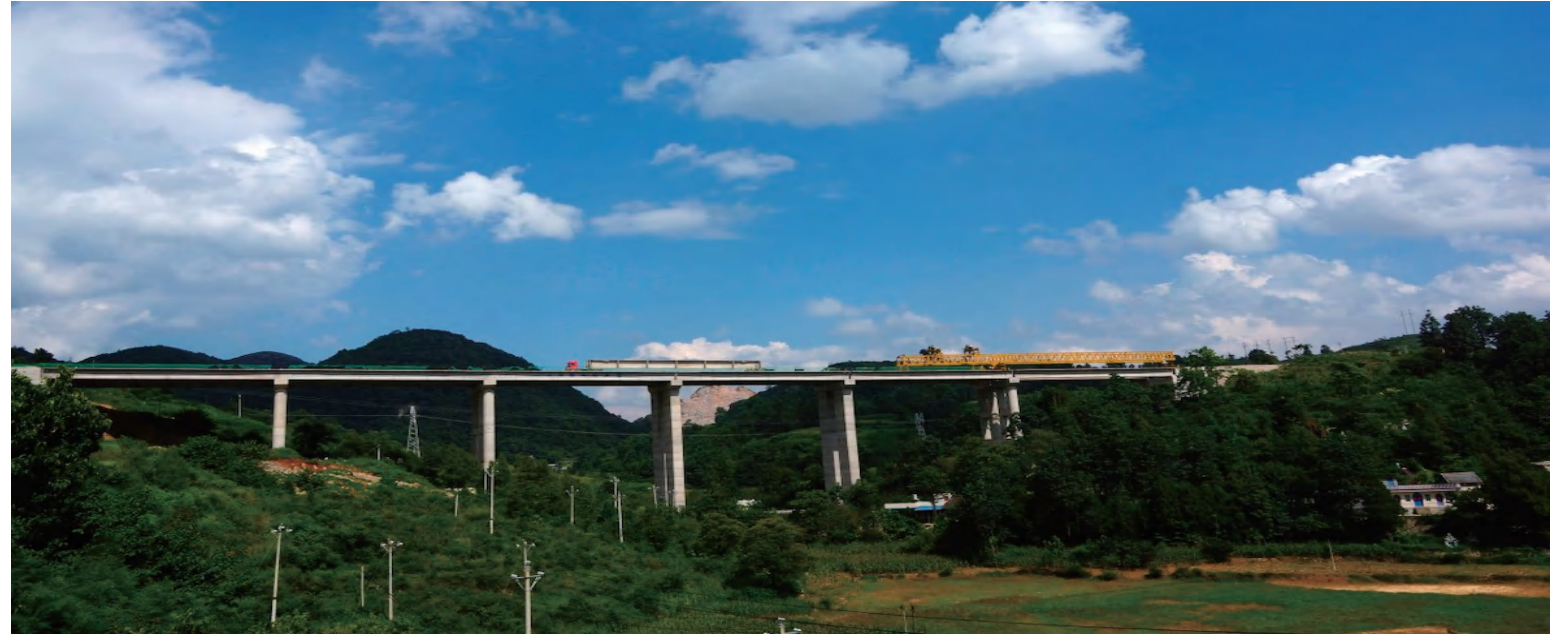
盘州快速路瓦窑田大桥 Wayaotian Bridge, Panzhou Expressway
