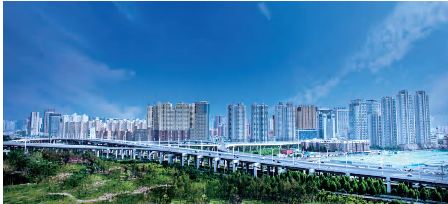
郑州农业路互通立交 Zhengzhou Agricultural Road Interchange
