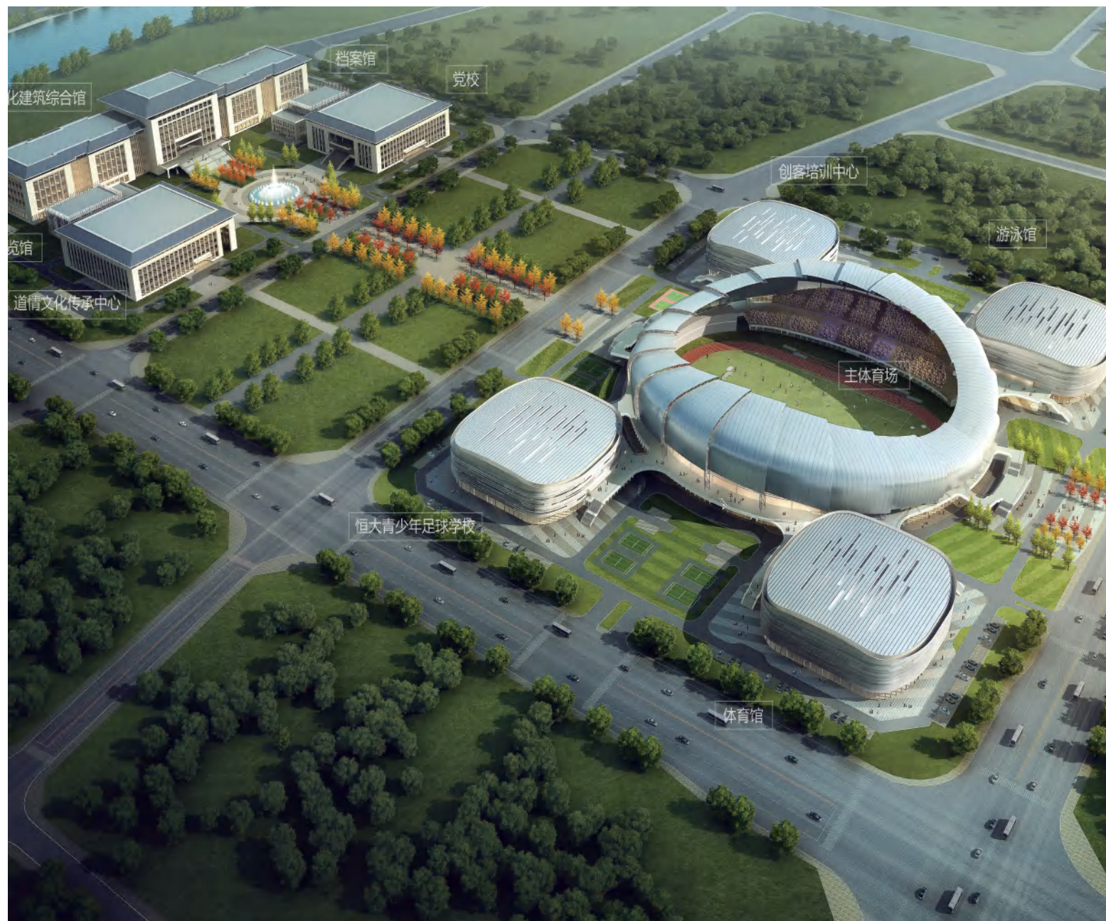
太康县党群综合服务中心建设项目 Construction project of party masses comprehensive service center in Taikang County
