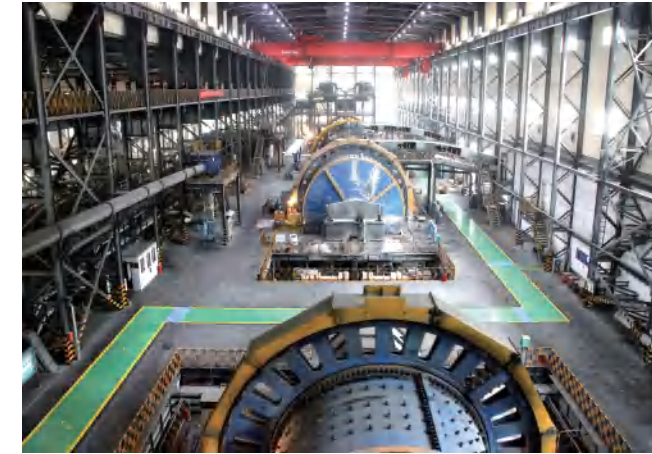
磨浮车间 Grinding and floating workshop
