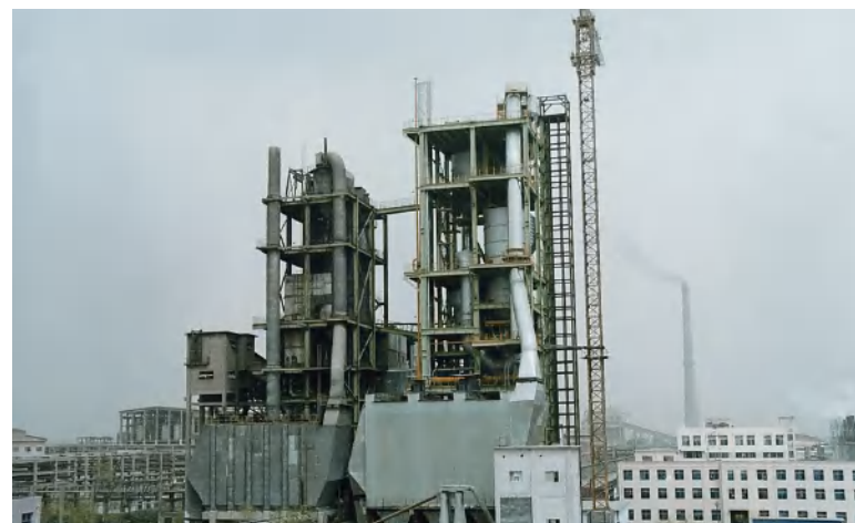
中铝山西新材料有限公司高压静电吸尘器 Aluminum Shanxi New Materials Co. LTD. High voltage electrostatic vacuum cleaner
