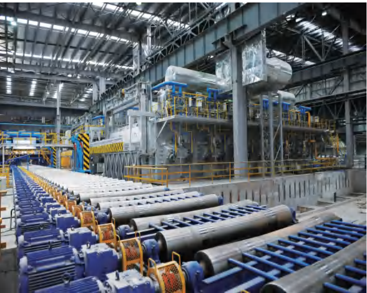
中铝瑞闽1+3连轧加热炉 Chalco Ruimin 1+3 continuous rolling furnace
