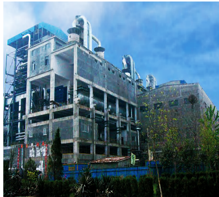
中州铝厂自配电厂 Zhongzhou aluminum plant with power plant
