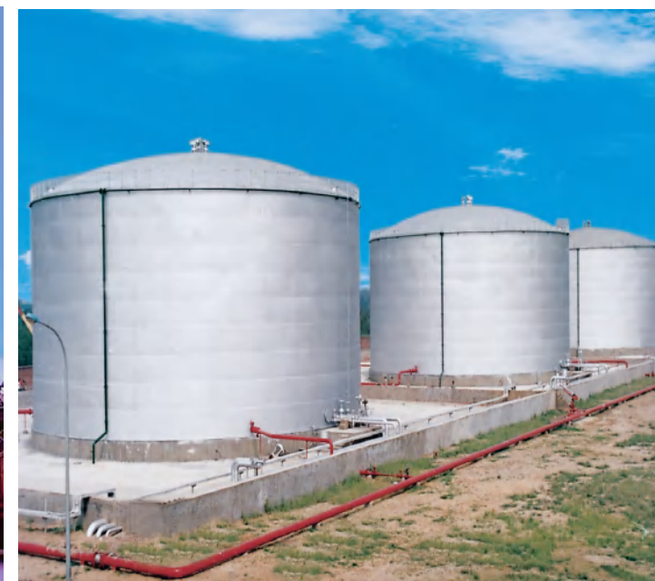
新郑机场10000立方米储油罐工程 Xinzheng Airport 10000 cubic meters storage tank project
