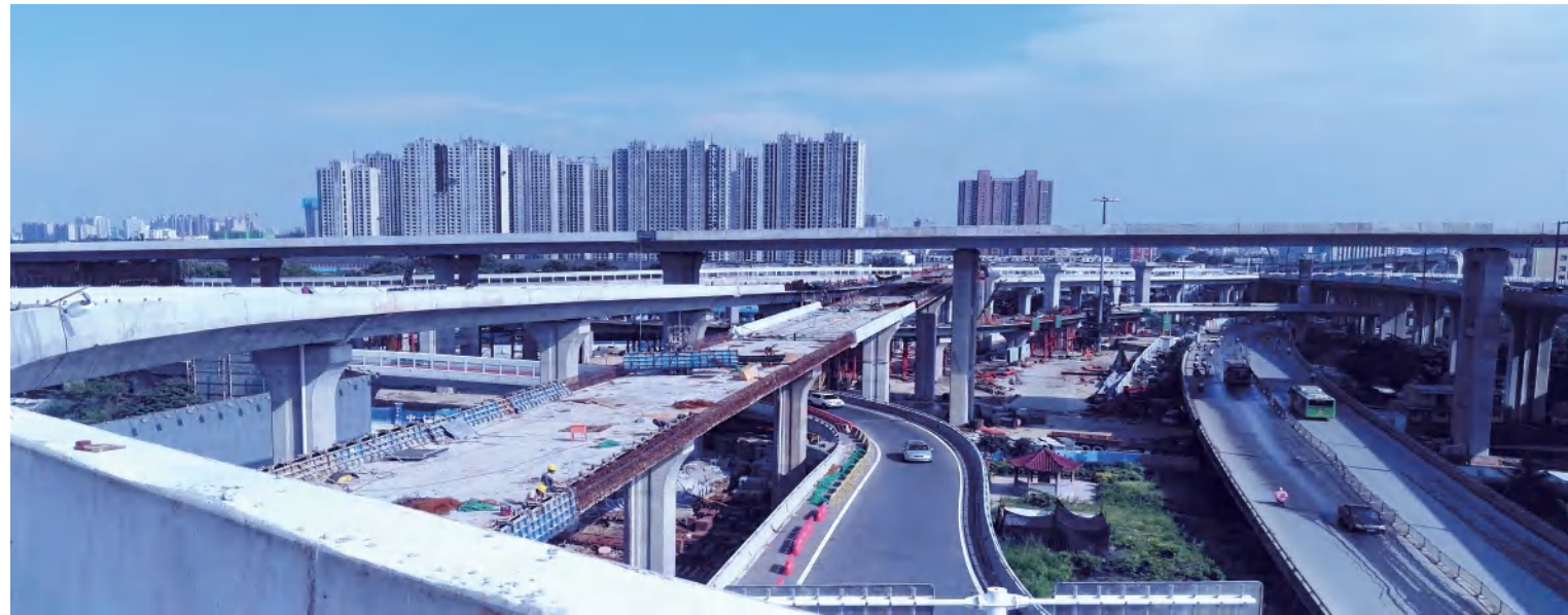
郑州农业路互通立交项目施工现场 Zhengzhou Agricultural Road interchange project construction site
