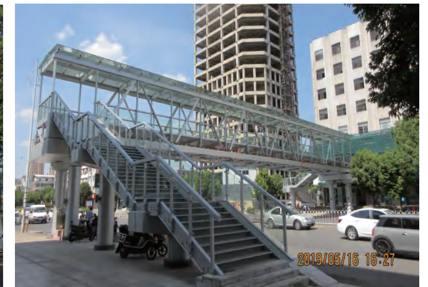
昆明市铝合金天桥 Kunming aluminum alloy overpass
