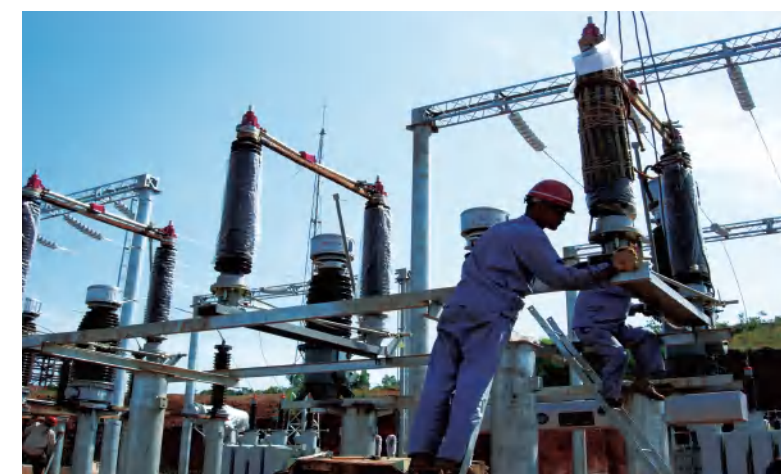
刚果（金）富利矿业公司变压器安装 Congo (DRC) Fuli Mining Company transformer installation
