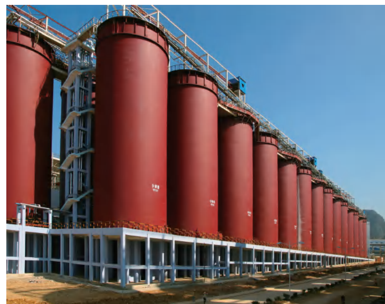
广西华银铝分解槽 Guangxi Huayin Aluminum decomposition tank
