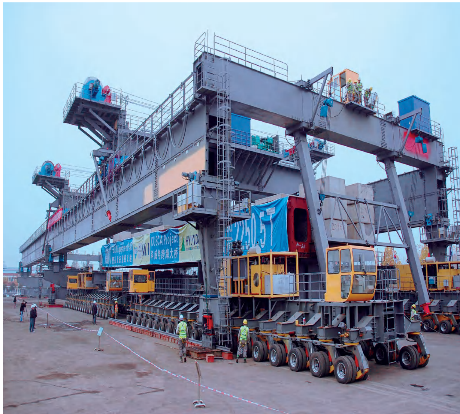
路桥设备--世界最大SDI1800架桥机 Road and bridge equipment -- the world's largest sdi1800 bridge erecting machine
