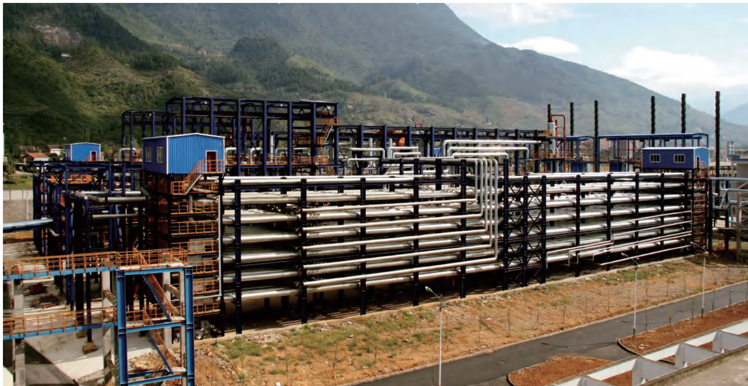
氧化铝项目高压溶出设备 Alumina project high pressure dissolution equipment
