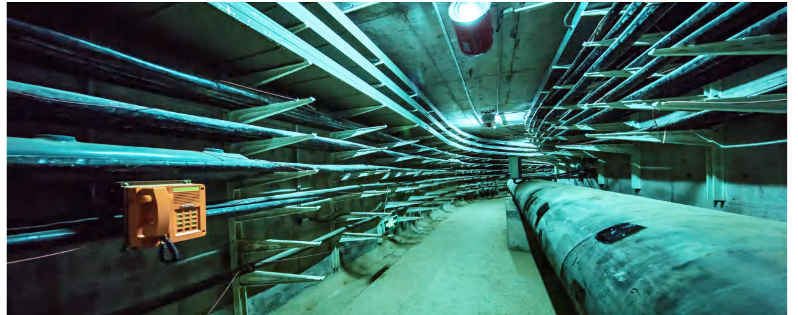
郑州航空港区地下综合管廊 Zhengzhou airport underground comprehensive pipe gallery
